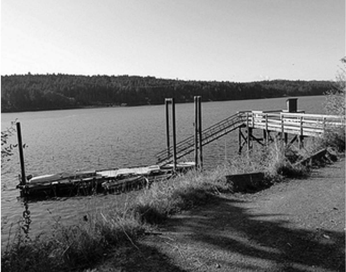
Green Wharf, December 19, 2011 after renovations.
