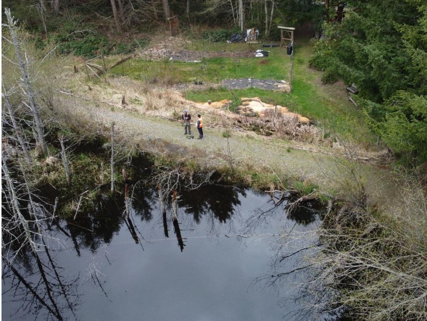
Photo 3-4 Existing earthen berm south of weir
