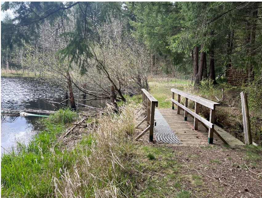
Photo 3-1 Wood bridge over Coats Creek and adjacent to cement weir
